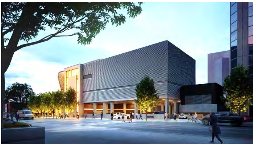
Edmonton's downtown district energy facility is in the Winspear Centre, shown here.
